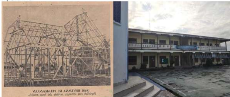
Figure 2 The renovated building in early 1952 and renovated building in 2017. Documentation 2018
