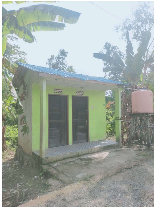
Gambar 4.38 Fasilitas WC PPS Sullamut Taufiq
