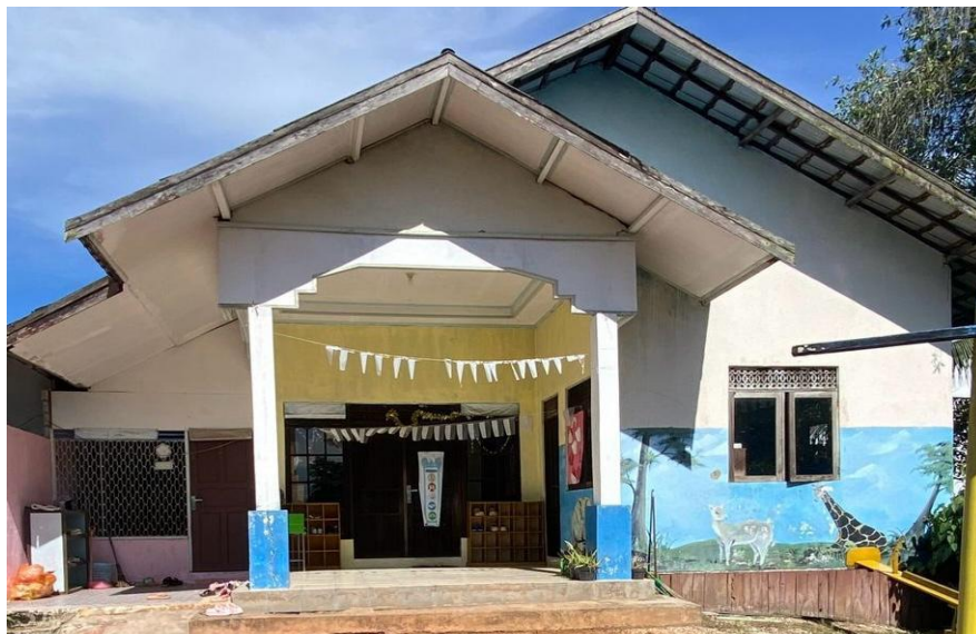
Gambar 4.1 Gedung PAUD Terpadu Riyadhus Sa'adah (CDGDFS.2.1) 1
